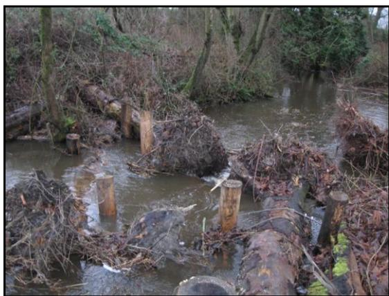
Large logs installed in Terrell Creek below the Kickerville Road culvert back water up to improve fish passage.
