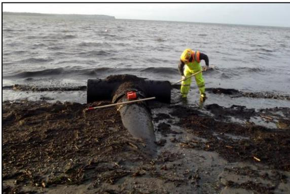
M&O staff cleaning a stormwater outfall pipe in Birch Bay.
