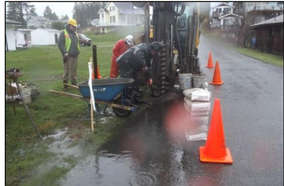
Boring holes for ground water monitoring wells in the Cottonwood project area.
