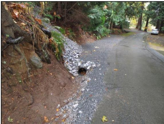
New stormwater pipe and catch basin system installed to carry stormwater flow from Semiahmoo Drive to Hogan Drive.
